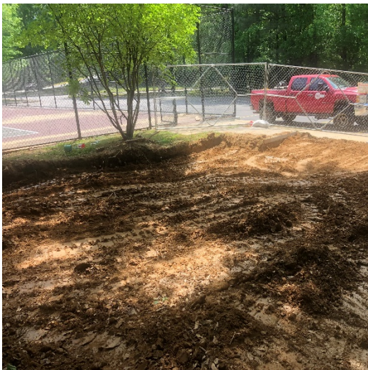
Backfill at Sanitary Tie-in
