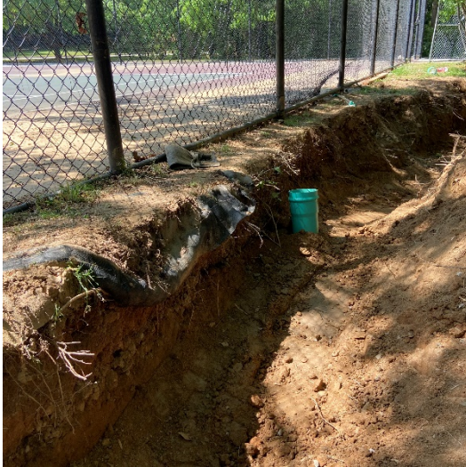
Sanitary Cleanout Install
