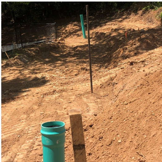
Sanitary Cleanout Install
